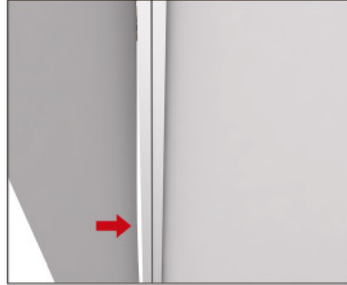
Step 14 Confirm all the fabric edges are pushed neatly and evenly into the horizontal and vertical profiles.
